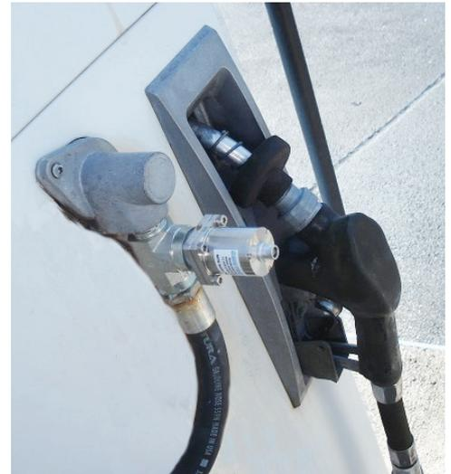
➤ Example of a DEVIL installation for in-line monitoring of fuel density on a fuel dispensing pump.
