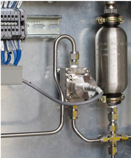
Figure 2. Example of NORTHDOME® integration into Wobbe index.
